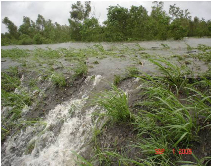
Figure 5: Close-up photograph of levee overtopping in Braithwaite, Louisiana during Hurricane Gustav.
