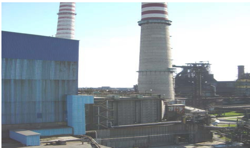
Figure 1: General view of the Mittal Steel Poland Power Plant in Krakow.
