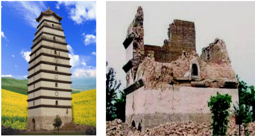
Figure 10: Wenxing pagoda: (left: before the earthquake; right: after the earthquake).
