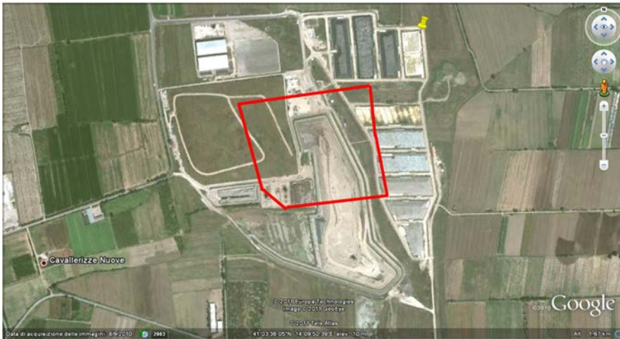
Figure 1: Satellite view of the Technological Pole area.
