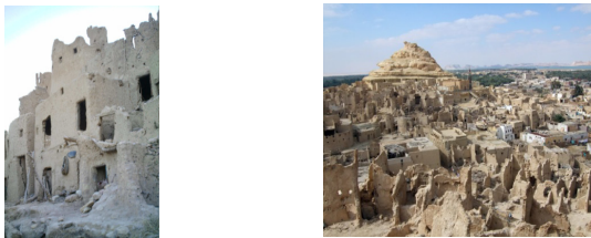
Figure 2: Ruins of the city of Shaly in which kerchief material was used in construction.
