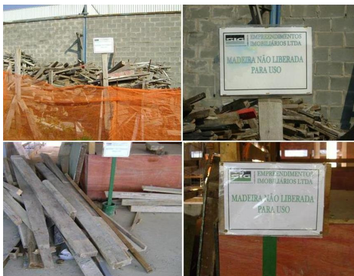
Figure 6: Wood separated for subsequent recycling processes.
