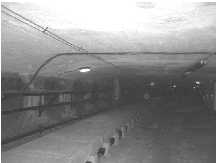
Figure 5: Queensway Tunnel Deck Soffit – prior to repair, approximately 60 years old (top) and 20 years after repairs were completed (bottom).
