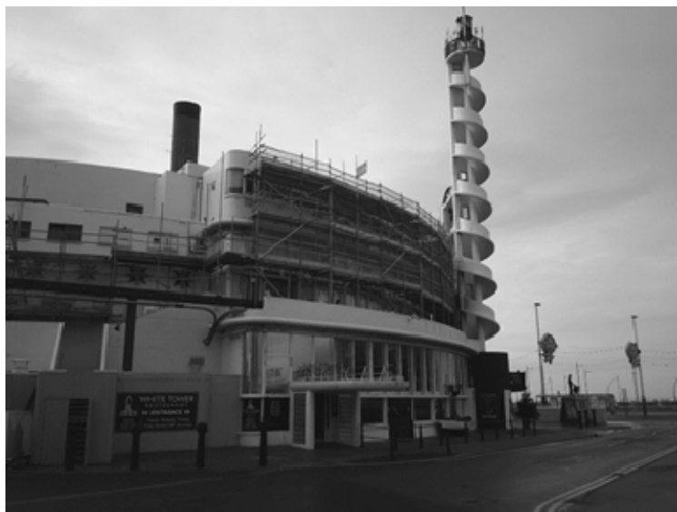
Figure 6: The White Building, Blackpool, during refurbishment.
