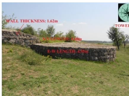
Figure 10: Dimensions of the circular tower “C” and E-W wall (Sucidava fortress, on Danube) (photo: A.B. Carlan, October 2013).
