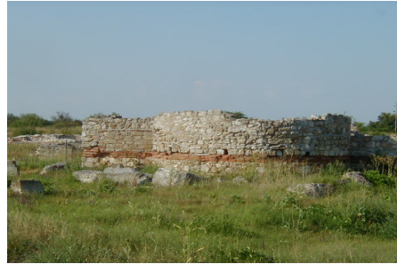
Figure 5: Defence walls and circular tower at Ulpia Oescus (photo: D. Constantinescu, August 2013).
