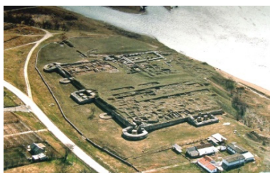
Figure 8: Castrum Capidava, aerial view, August 2002.
