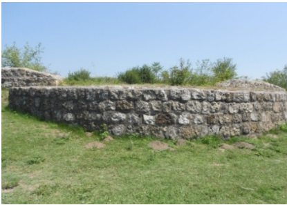
Figure 4: Defence wall and circular tower at Sucidava sites (photo: D. Constantinescu, August 2013).
