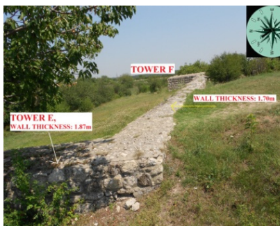
Figure 11: Defence wall and towers “E” and “F” (Sucidava fortresses, on Danube) (photo: A.B. Carlan, October 2013).
