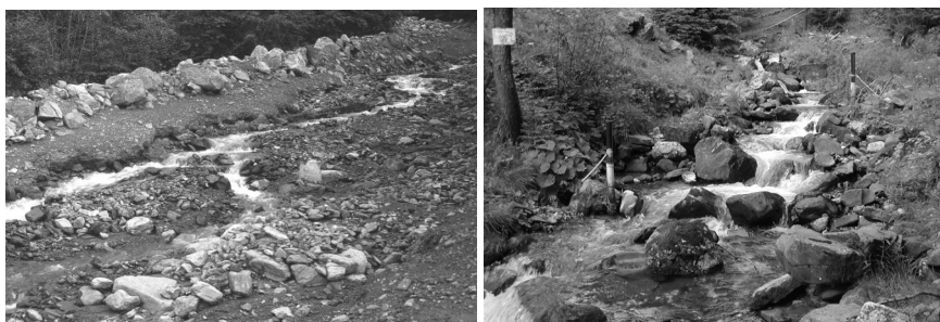
Figure 2: Pictures of the Moscardo Torrent (left) and the Rio Cordon (right) main channels.
