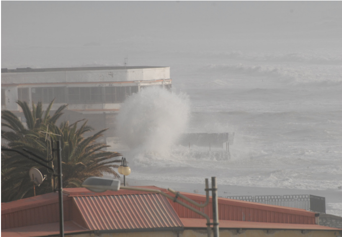
Figure 3: Storm surge and wave-induced damage to buildings during the winter 2008 storms.
