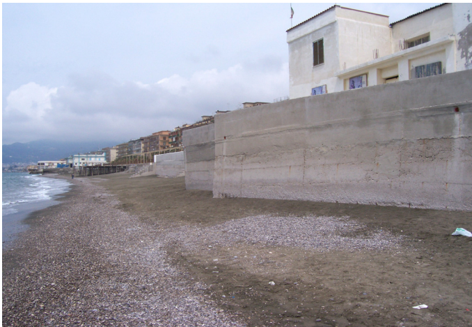
Figure 1: Salerno inhabited coastline protected by a vertical wall without any defence work.
