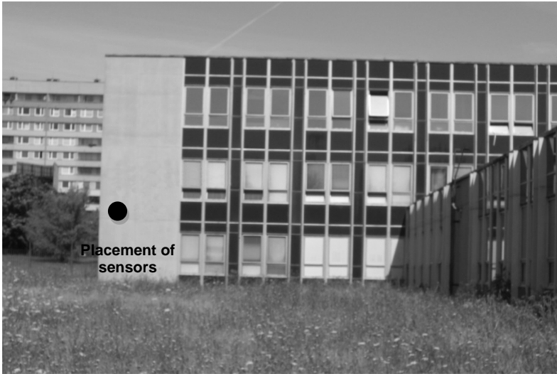
Figure 2: View of the studied building and sensor placing.
