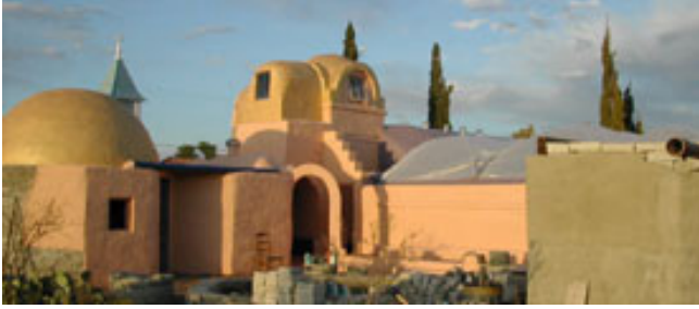
Figure 3: Papercrete domes and vaults built without interior reinforcement.
