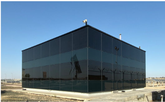
Figure 1: The CUBE BIPV test facility at DEWA R&D center. (Source: Photo by authors.)
