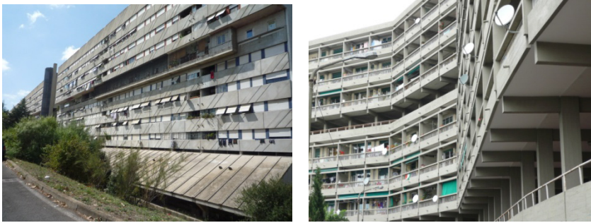
Figures 1-2: Social housing stocks in Italy: Corviale in Rome and Forte Quezzi in Genoa.
