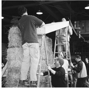
Figure 5: Strawbale mock-up wall.
