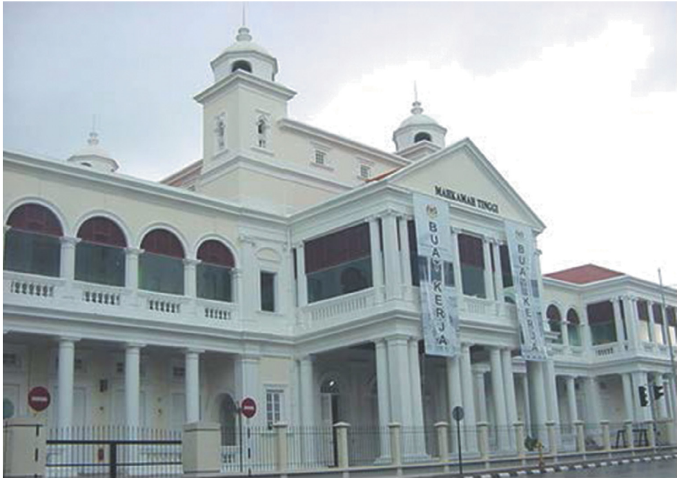
Figure 3: High Court Building.
