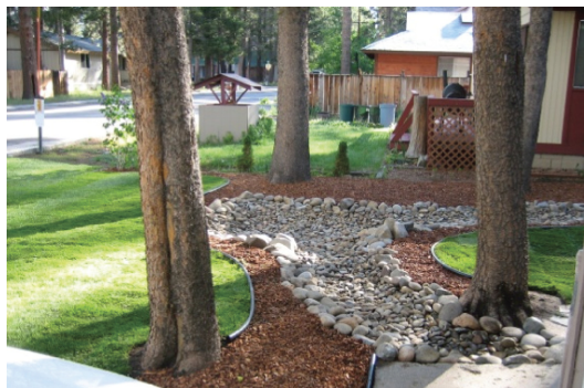
Figure 8: This infiltration basin will store roof runoff until it can percolate into the ground [3].
