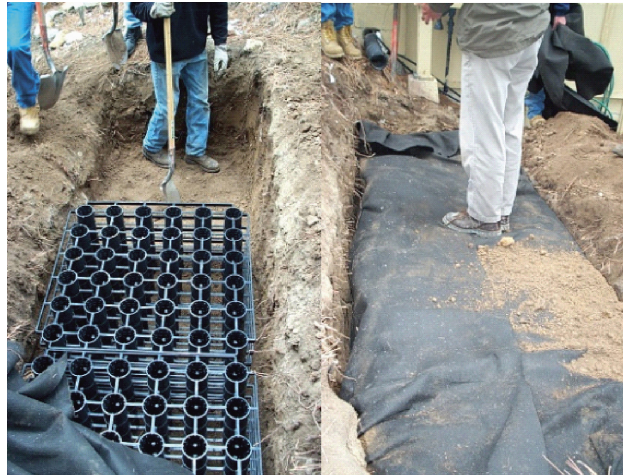
Figure 6: Infiltration systems filled with prefabricated storage units store more water than those filled with gravel. The tops and sides are wrapped with filter fabric and covered with gravel [6].
