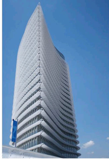
Figure 41: The Water Tower, 2008, Zaragoza.
