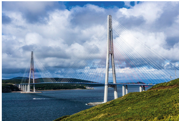
Figure 10: Russky Island bridge.
