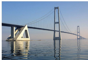
b) Great Belt bridge
