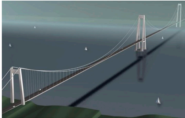
Figure 16: Chacao bridge (Chile).
