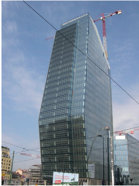
Figure 36: Diamond Tower, Milan (140 m), 2012.
