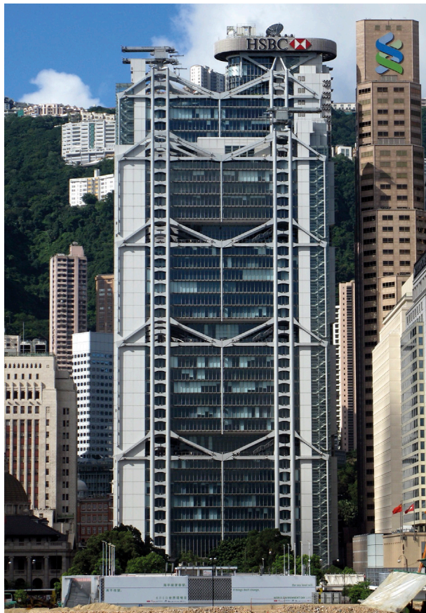
Figure 20: HSBC building, Hong-Kong.
