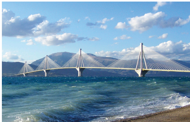
Figure 13: Rion-Antirion bridge (Greece).
