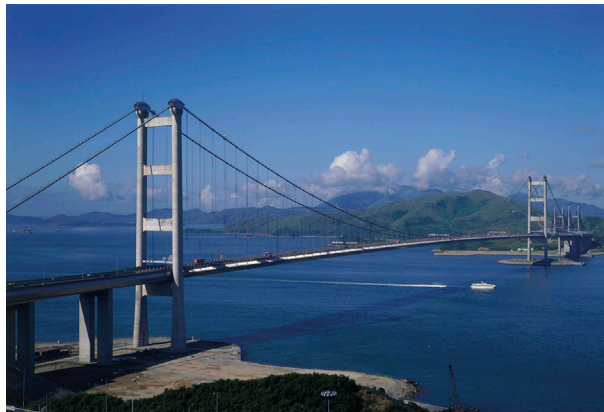
Figure 5: Tsing Ma bridge.
