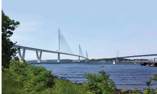
Figure 15: Queensferry Crossing (UK).
