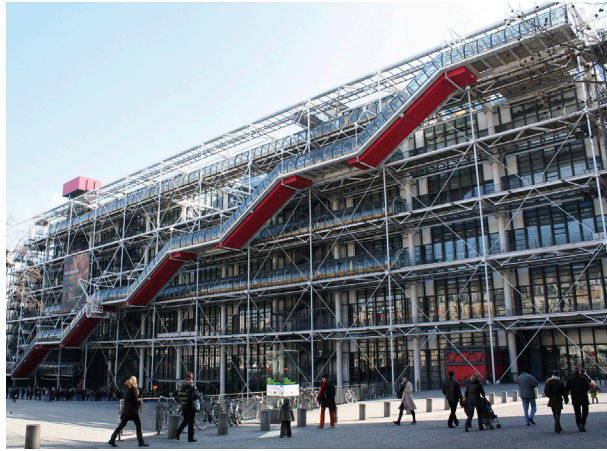
Figure 19: Pompidou Centre, Paris.
