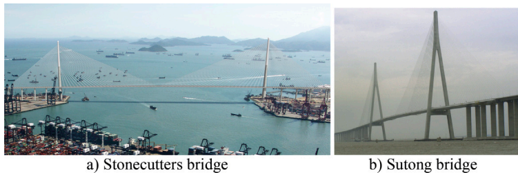
Figure 8: Cable-stayed bridges in China.
